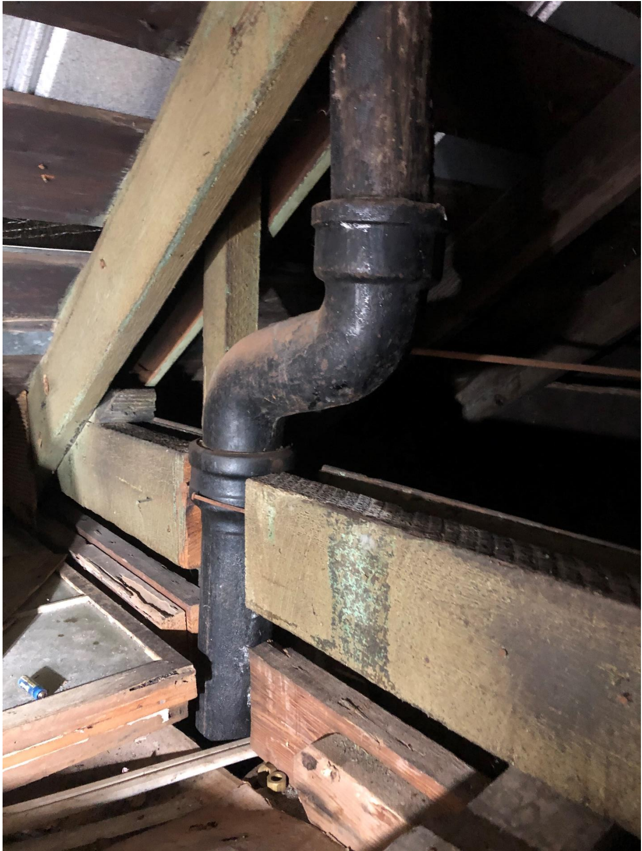
Ceiling joists and collar ties cut through in a few locations
