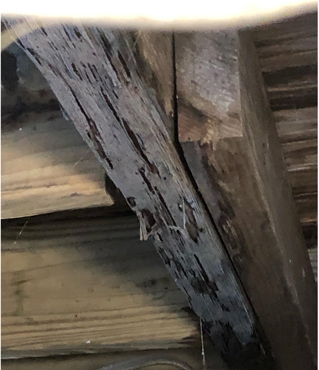
Floor joists are termite infested
