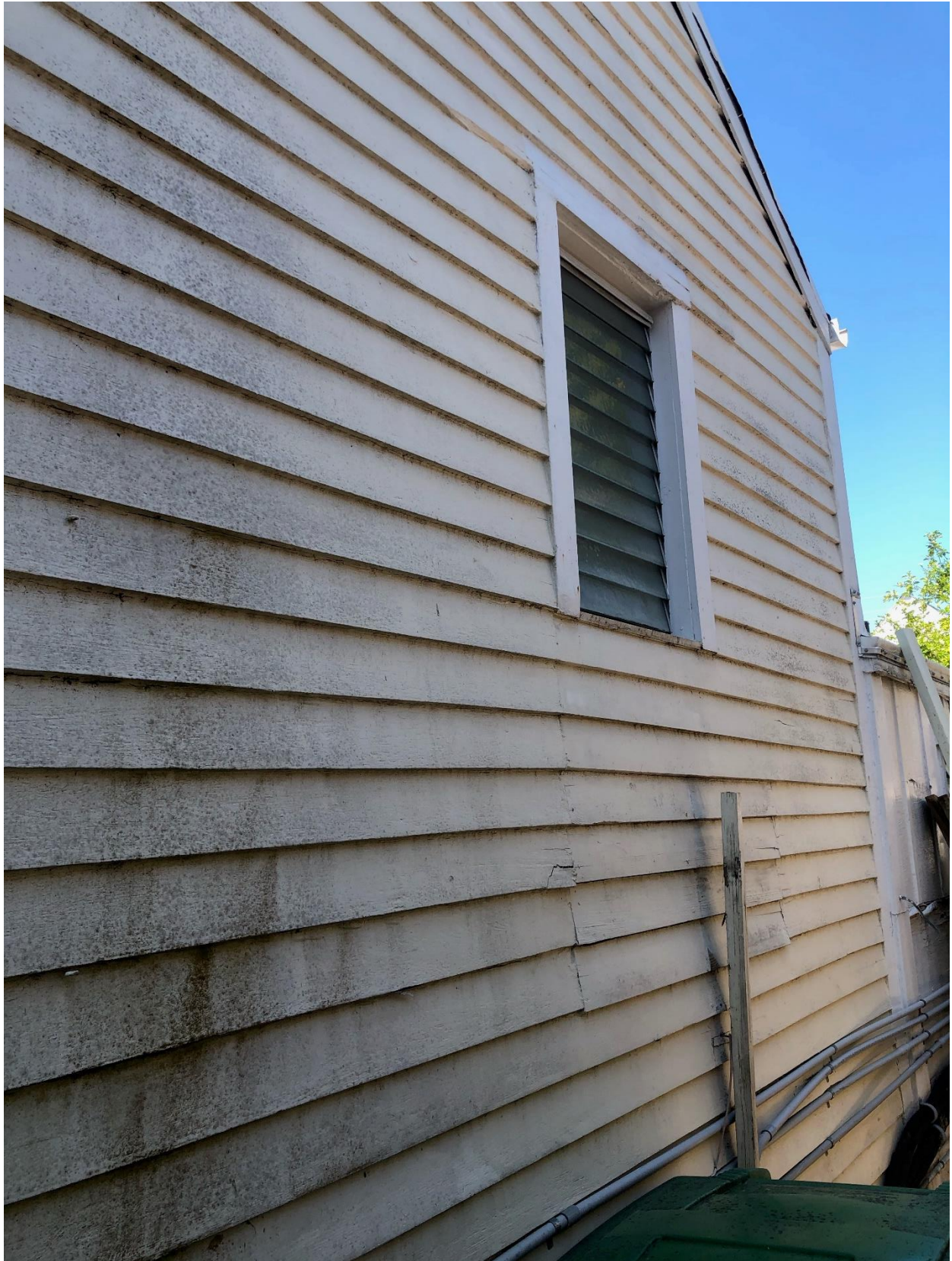
Trim does not match on the sawtooth addition
