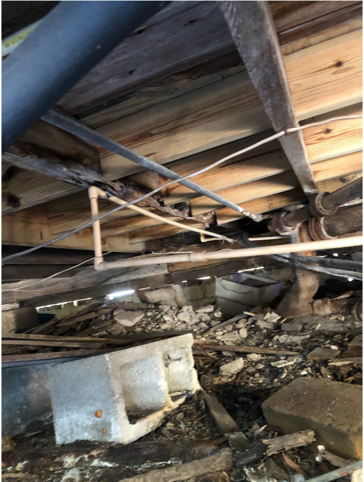
New framing is just blocking not adding strength
