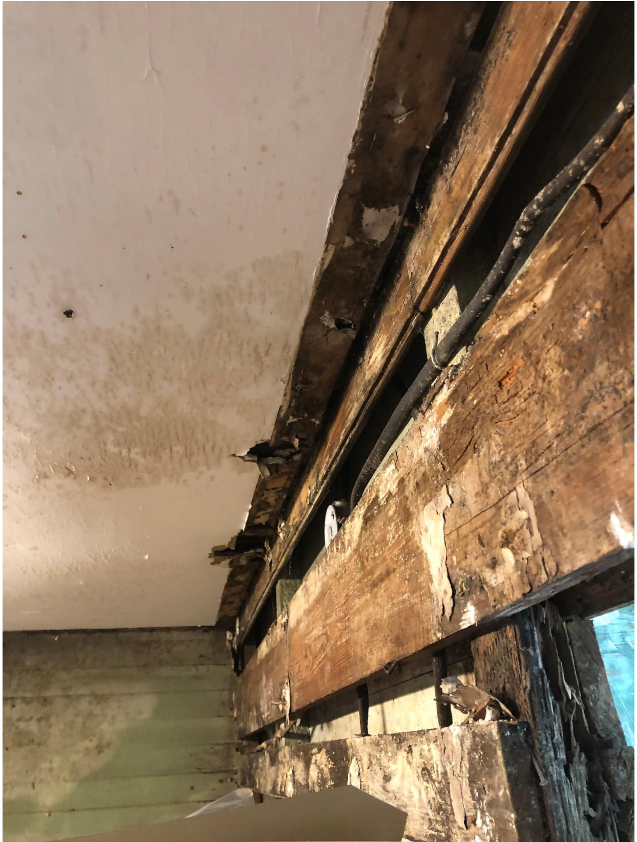
Interior framing has water damage, sheetrock ceiling has mold
