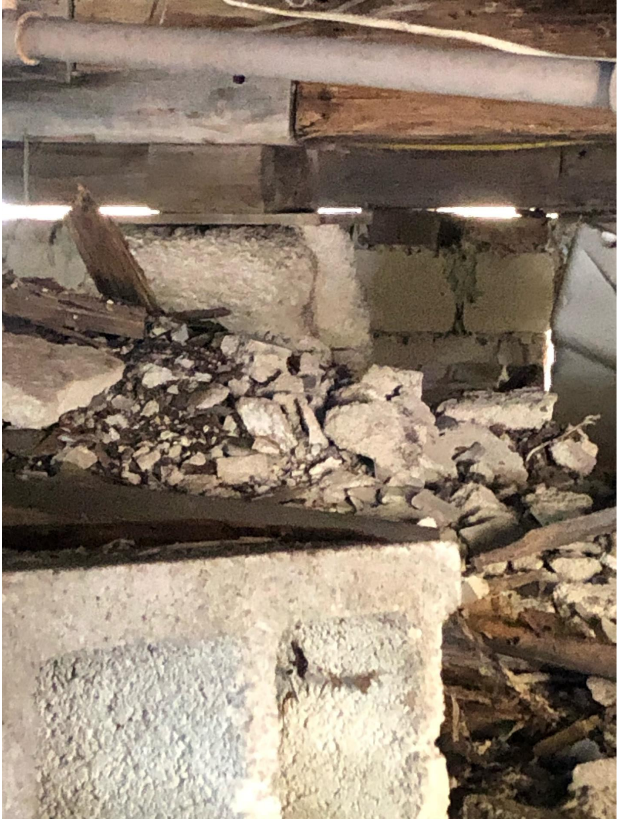
Foundation in rear sawtooth is not strong and different materials used
