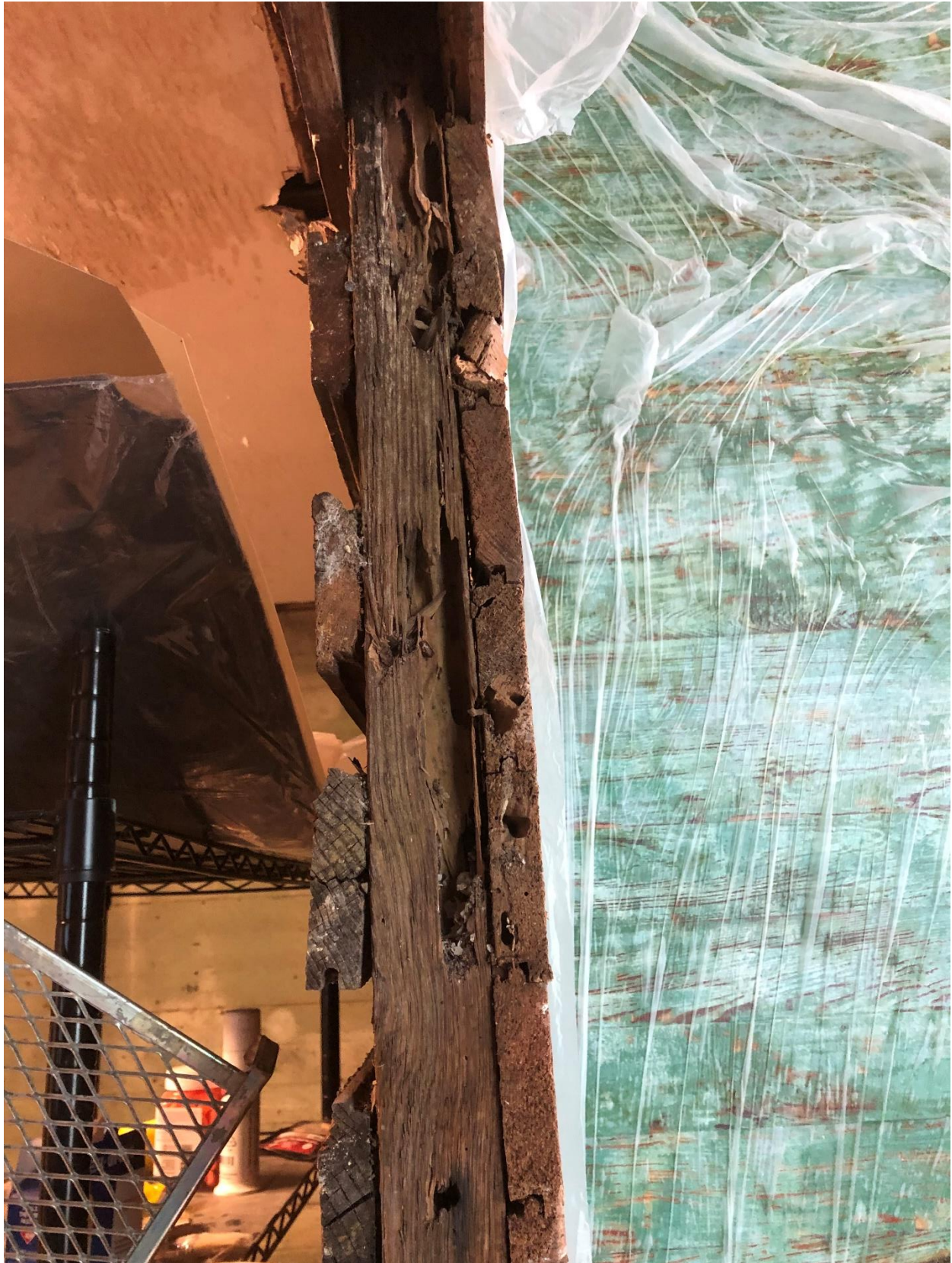
Interior wall framing is rotten, mold on ceiling
