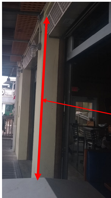
Figure 24. Location 24: Approximately 10 ft long new 16x12 concrete column. See detail 6/S104.
