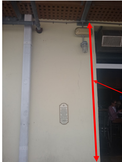
Figure 24. Location 24: Approximately 10 ft long new 16x12 concrete column. See detail 6/S104.
