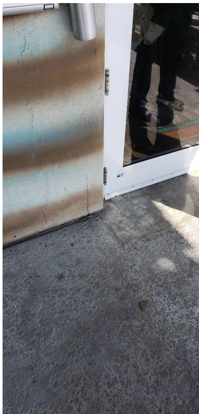
Figure 12. Front Entrance. Location 12: 8x8 cell of the end CMU block to be fully grouted from header to ground.
