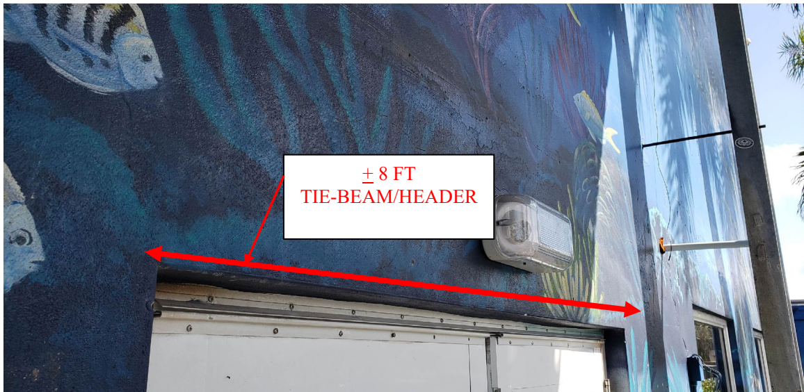
Figure 12A. Front Entrance. Location 12: 8 ft long new tie-beam/header. See typical detail 8/S105.
