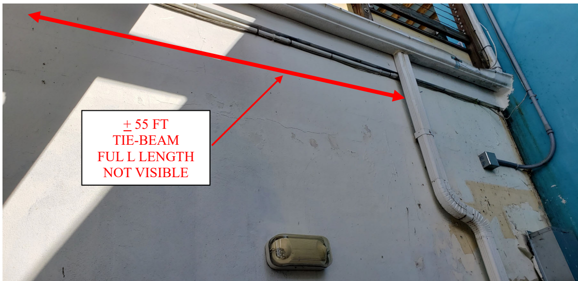
Figure 5. Location 5: Approximately 55 ft long new 12x24 horizontal tie-beam. See detail 3/S103.
