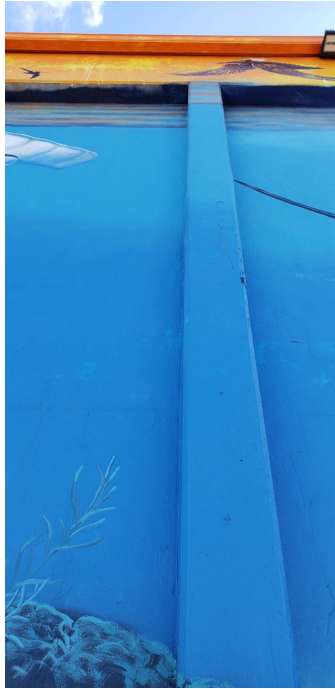
Figure 9. Location 9: Approximately 26 ft long new 12x16 concrete column. See detail 2/S102.
