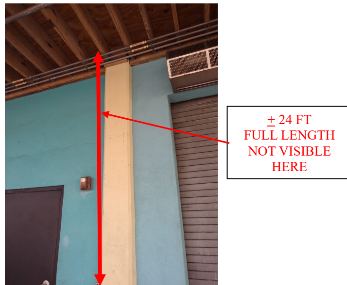
Figure 16. Location 16: Approximately 24 ft long new 12x12 concrete column. See detail 2/S102.
