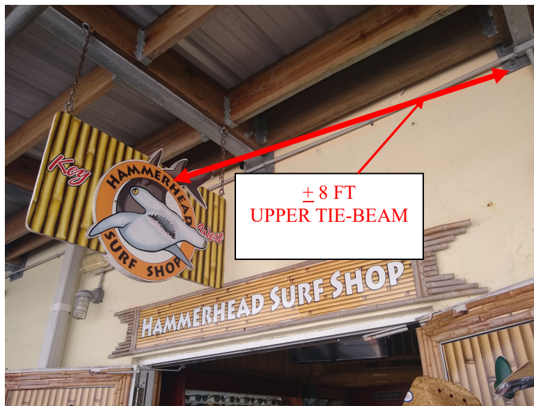
Figure 28A. Surf Shop. Between Location 28 and 29: Approximately 8 ft long new 8x16 horizontal tie-beam. See detail 5/S104 - tie-beam / header replacement detail.
