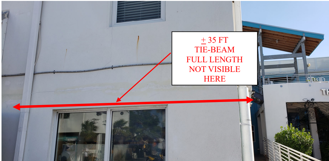
Figure 34. Location 34: Approximately 35 ft long continuous new 8x16 horizontal tie-beam/header above opening. See detail 7/S105.
