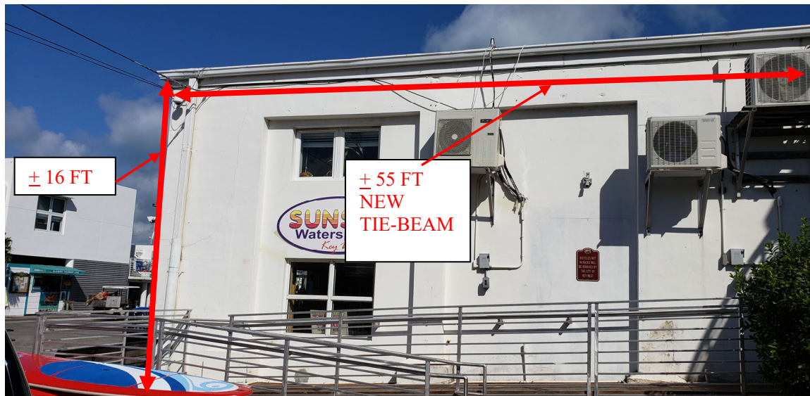
Figure 1. Front Elevation near roundabout. Location 1: Approximately 16 ft long new corner 16x12 concrete column. See detail 1/S101. Approximately 55 ft long new 12x24 horizontal tie-beam. See detail 3/S103.
