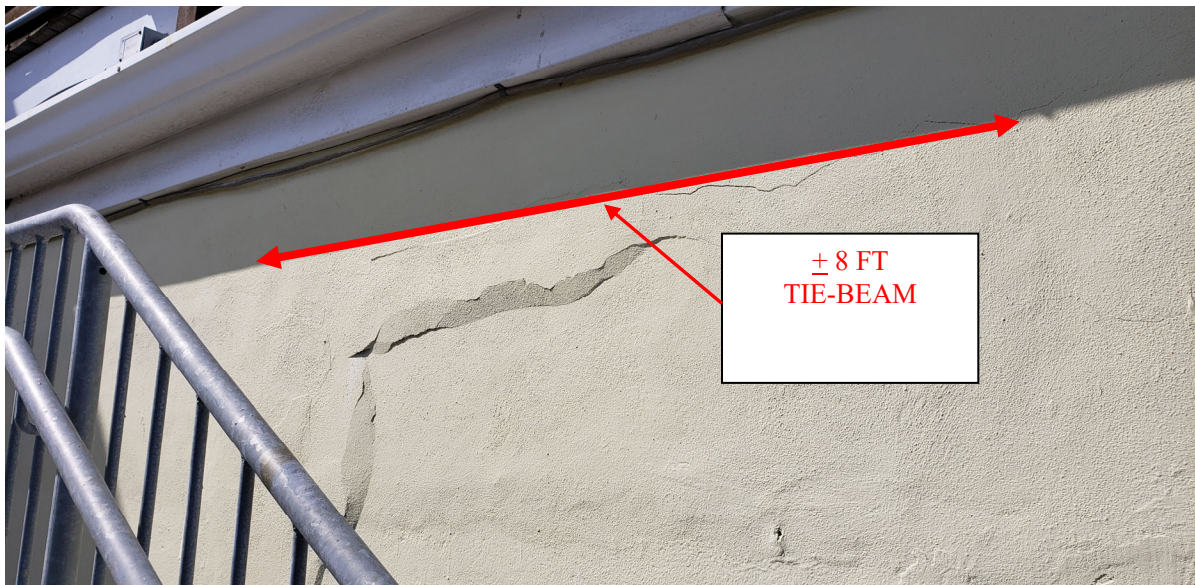
Figure 21A. Between Location 21 and Location 22. Approximately 12 ft long new 8x16 horizontal tie-beam. See detail 5/S104.
